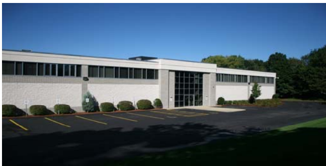
Building Section C – 1 st Floor (160' x 219'9") 35,000 SF - 2 nd Floor (160' x 124') 19,840 SF - 3 Loading Docks
